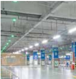
Indoor structures, underground parking area
