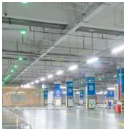
Indoor structures, underground parking area
